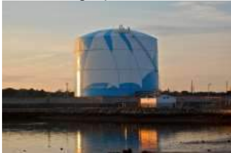
Şekil 5. A liquefied natural gas storage tank in Massachusetts.
