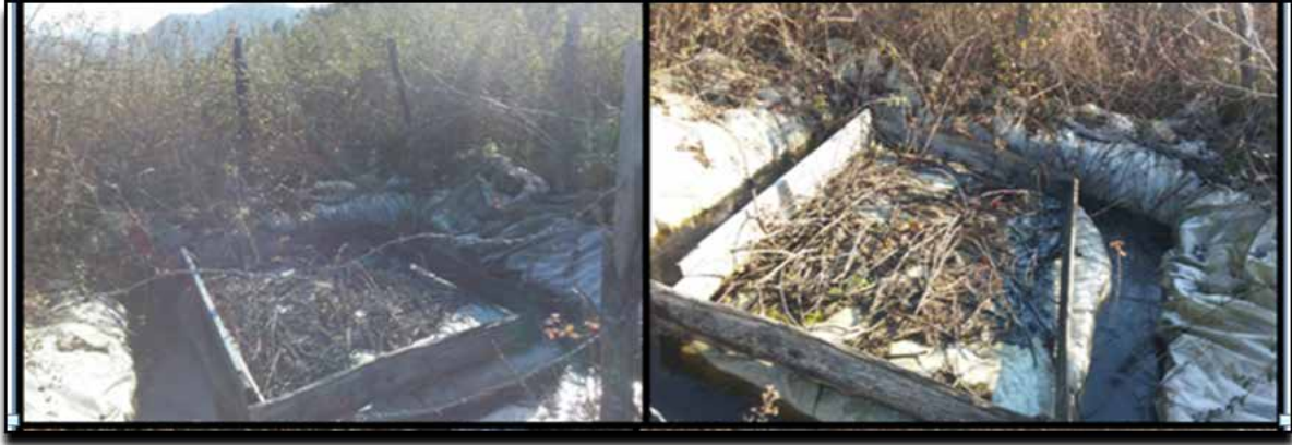
Figure 9. The islet area prior to restoration (SOBUTAY, U., 2014)
